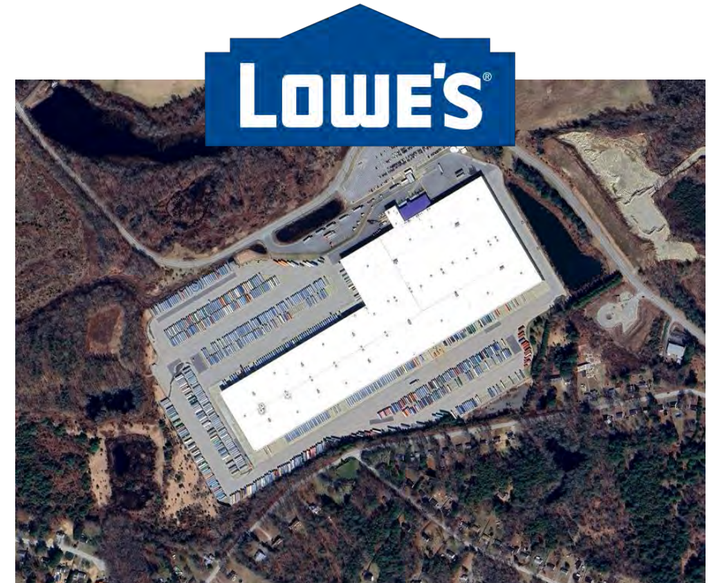
Lowe's Distribution Center Plainfield Image: Google Maps
