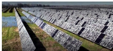
Solar panels damaged by hail in March 2024 in Needville, TX at a 350 MW solar farm
