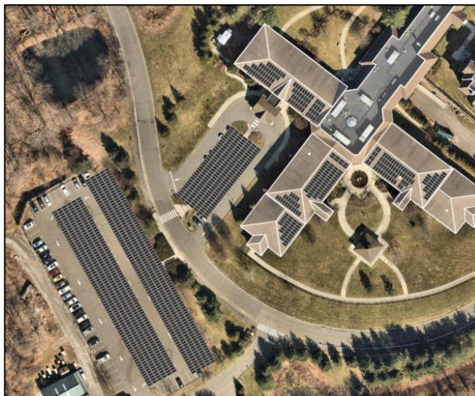
Photo 1. Overhead View (provided by contractor)
