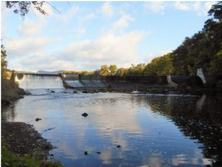
No. 2 Overview of dam from downstream.
