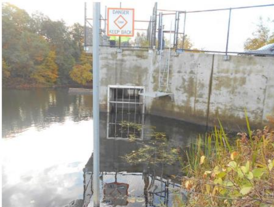
No. 10 Upstream end of fishway at the right training wall.
