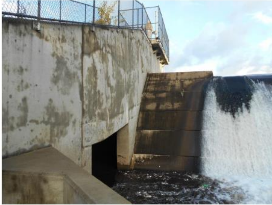
No. 7 Outlet structure through the right training wall below the fishway.
