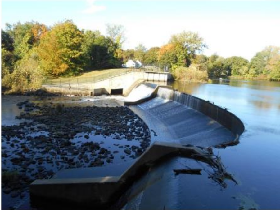
No. 1 Overview of dam from left abutment.
