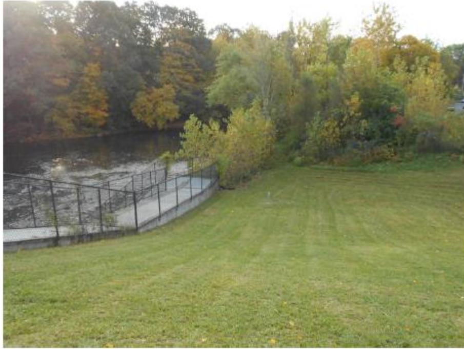
No. 11 Downstream embankment of dam at the right side.
