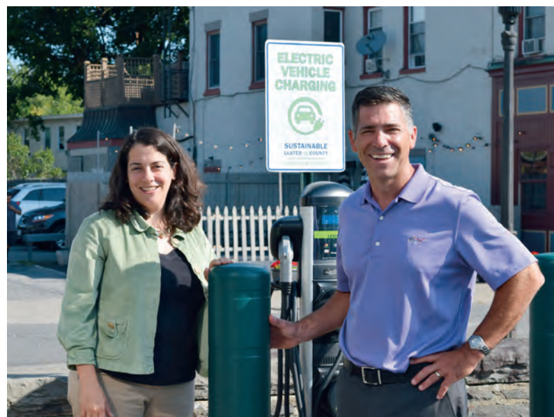
The first Clean Energy Community designated in New York was Ulster County. Amanda LaValle and Mike Hein stand next to the EV charging station the County installed as part of the Clean Energy Communities Program. Source: County of Ulster.
