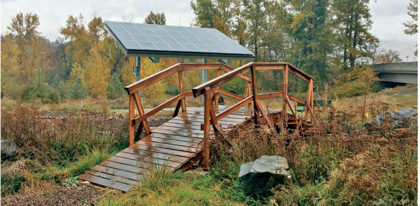
This solar array at Coyote Trails School of Nature in Medford, OR was awarded $11,356 in RED Grant Program funds by the Oregon Department of Energy. Source: Jennifer Kalez, Oregon Department of Energy.
