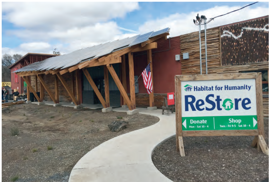
This solar array at Bend Area Habitat for Humanity ReStore received awarded $36,120 in RED Grant Program funds by the Oregon Department of Energy. Source: Jennifer Kalez, Oregon Department of Energy.
