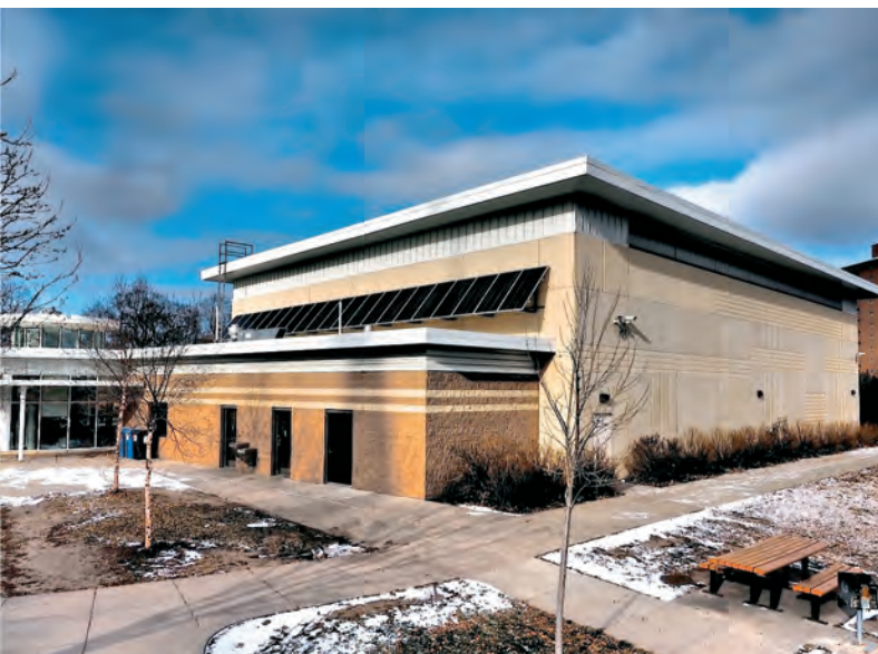
A 6.5-kW wall-mounted array at the East Phillips Park Community and Cultural Center in Minneapolis. Source: Ray Colby/Sundial Solar.
