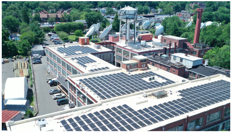
With a roof covered with solar panels, the Glenbrook Industrial Park in Stamford is home to a number of artisans, makers and light manufacturers.
