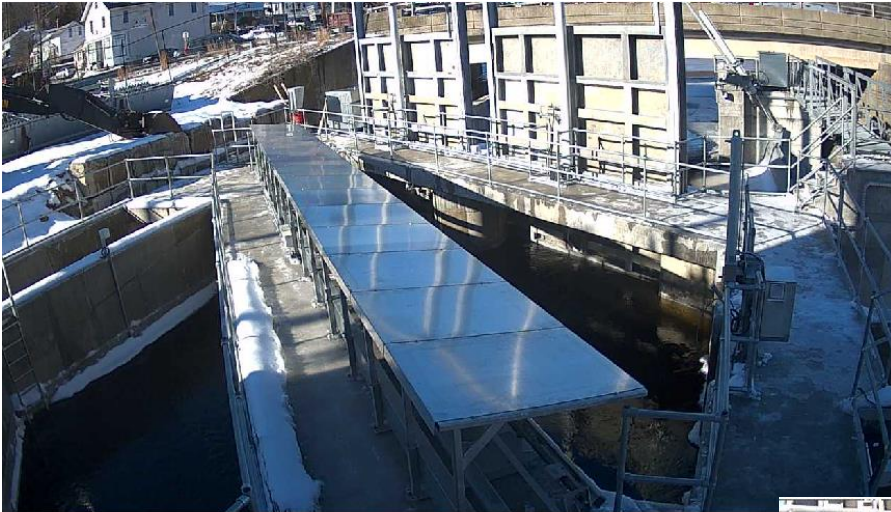
Inlet and gates
