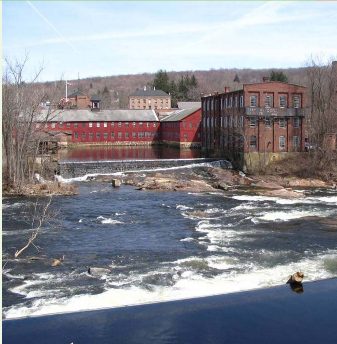
The historic powerhouse at the Upper Collinsville Dam on the Farmington River in Canton will produce 1 MW of hydroelectric power when restoration is complete.
