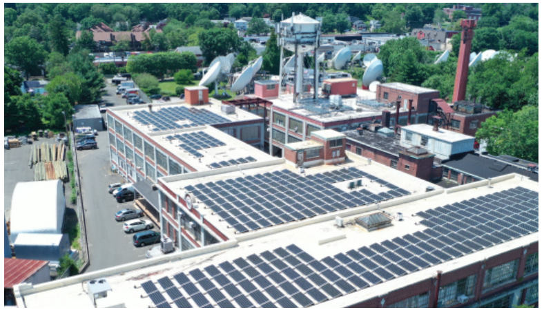
With a roof lined with solar panels, the Glenbrook Industrial Park in Stamford is home to a number of artisans, makers and light manufacturing firms.
