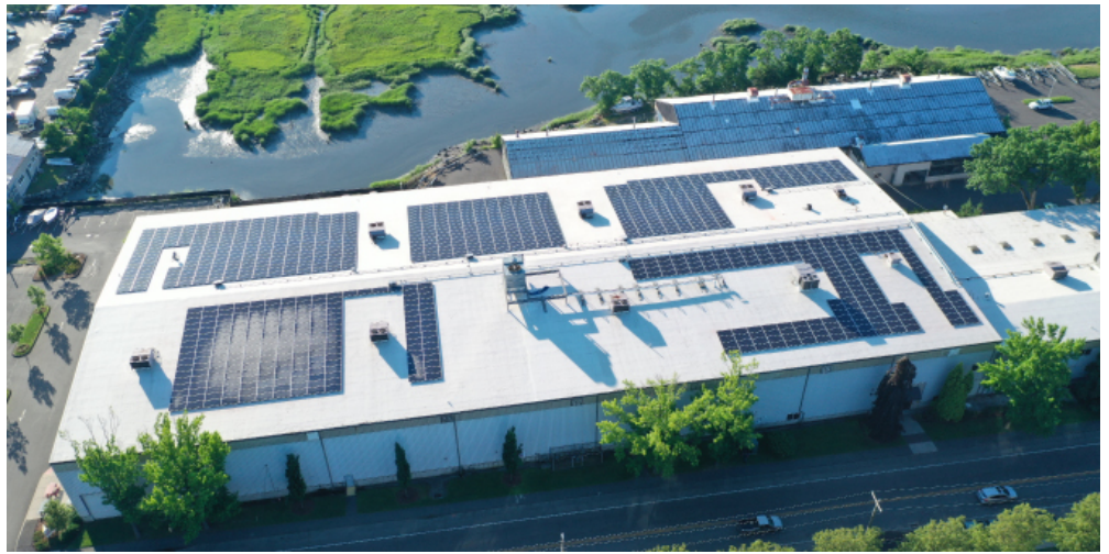
A drone photo of the solar PV system at the SoNo Ice House, a state-of-the-art facility featuring two ice skating rinks, in South Norwalk.
