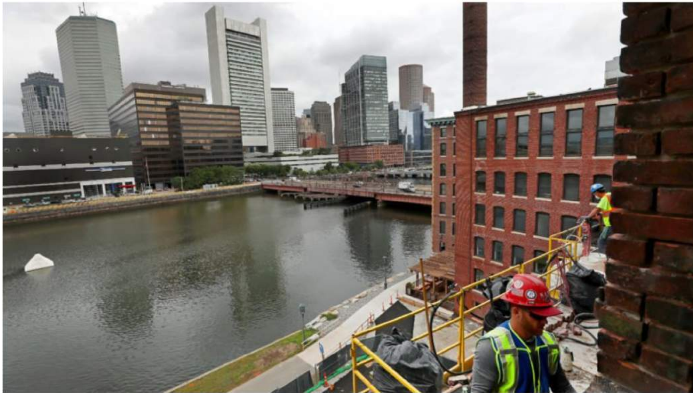
Work was underway in August on General Electric's Fort Point offices. —David L. Ryan/The Boston Globe
