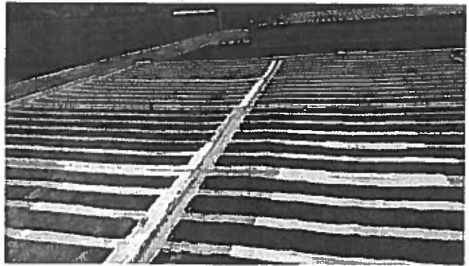
ALL COMBINER BOXES ARE "BURIED" IN ROOF SURFACE. ALL STRING WIRING FOR DC SOURCE CIRCUITS IS IN PVC CONDUITS BURIED IN ROOF SURFACE AND IS INACCESSIBLE. A CHECK OF THE INDIVIDUAL STRING VOLTAGES REVEALED THAT MANY IF NOT MOST STRINGS ARE OPERATING AT SEVERLY REDUCED VOLTAGES, WITH SOME "DEAD" CIRCUITS. SINCE ALL WIRING IS PERMANENTLY BURIED IN THE ROOF SURFACE, DIAGNOSIS AND REPAIR IS IMPOSSIBLE.
