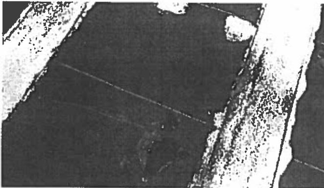
ENTIRE ARRAY HAS BEEN "PATCHED" AND RE-FASTENED TO ROOF SURFACE USING A SYSTEM OF GAUZE AND SEALANT AFTER MODULES HAD BEEN SEVERLY DELAMINATING FROM ROOF SURFACE AND REPORTEDLY CAUSING LEAKS. THIS RESULTED IN COVERING OF THE EDGES OF THE PV MODULES AND PARTIALLY BLOCKING THE CELLS ON EVERY MODULE.
