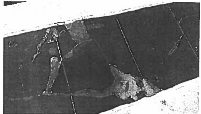
EXAMPLE OF DAMAGED PROTECTIVE LAYER AND EXPOSED CELLS
