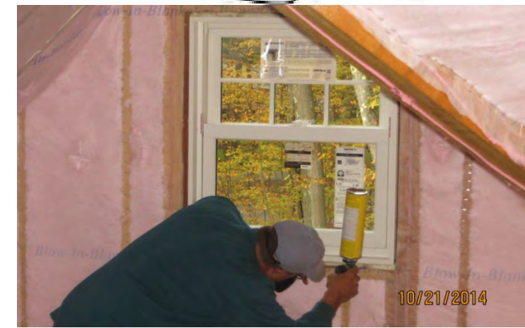
Air sealing during construction
