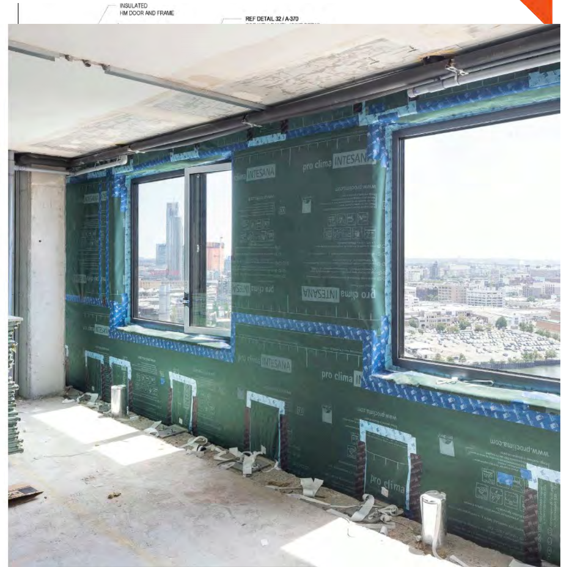
Air Barrier Installed
