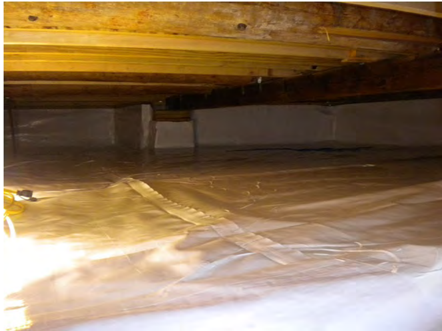
Existing · Crawl Space
