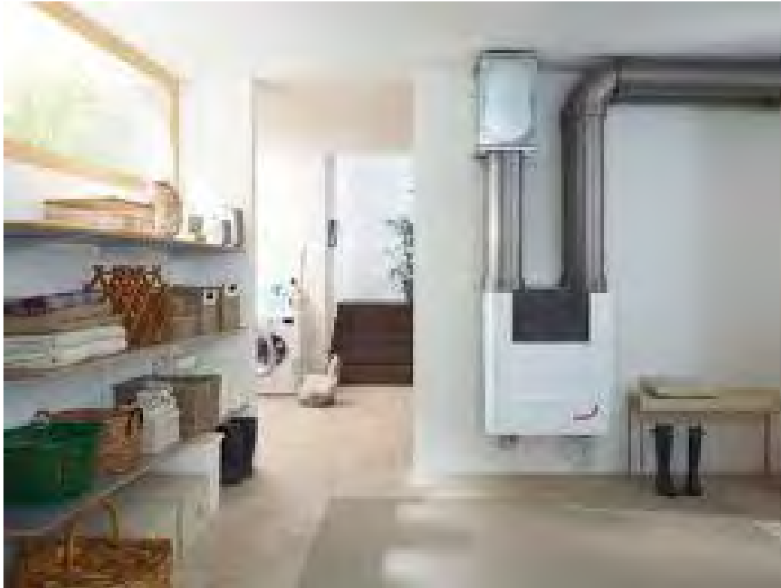
Energy Recovery Ventilation
