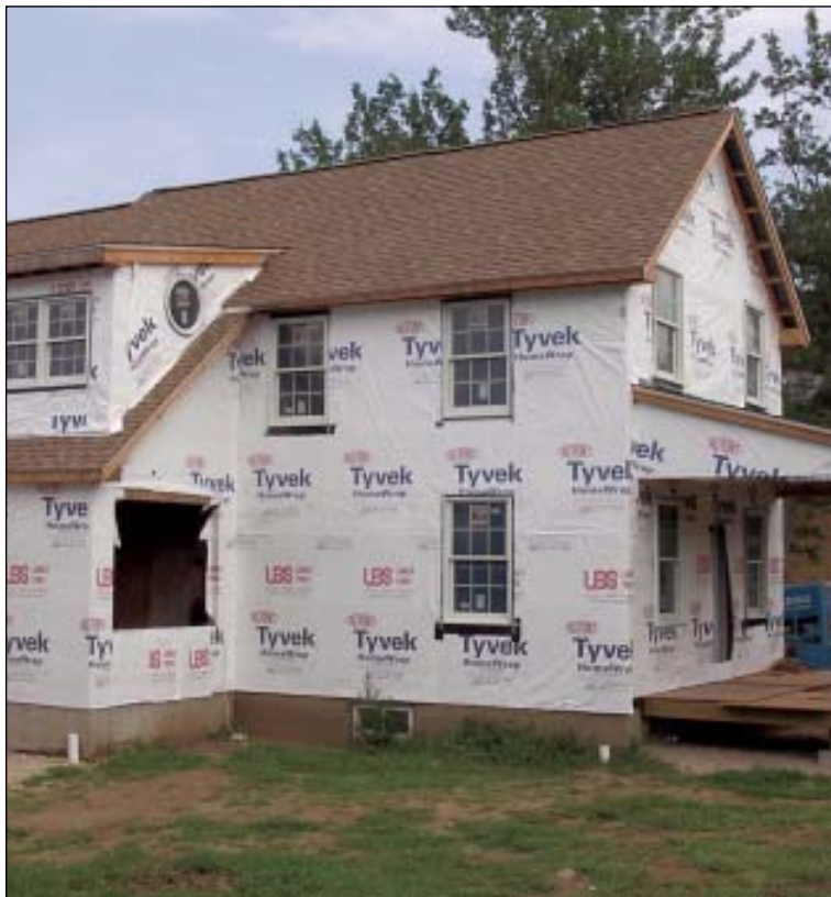
FIGURE 3. Contractor Craig Caulkins of Caulkins Building & Design in Niantic, Conn., routinely applies 1/2-inch or 1-inch Dow Styrofoam to home exteriors under vinyl siding (above right). While foam is water resistant and provides a good barrier against the bulk of the weather, wind-driven rain can find its way around panels and through joints, so Caulkins relies on a housewrap and careful window flashing installed over a fully sheathed structure before installing the foam (above left).
