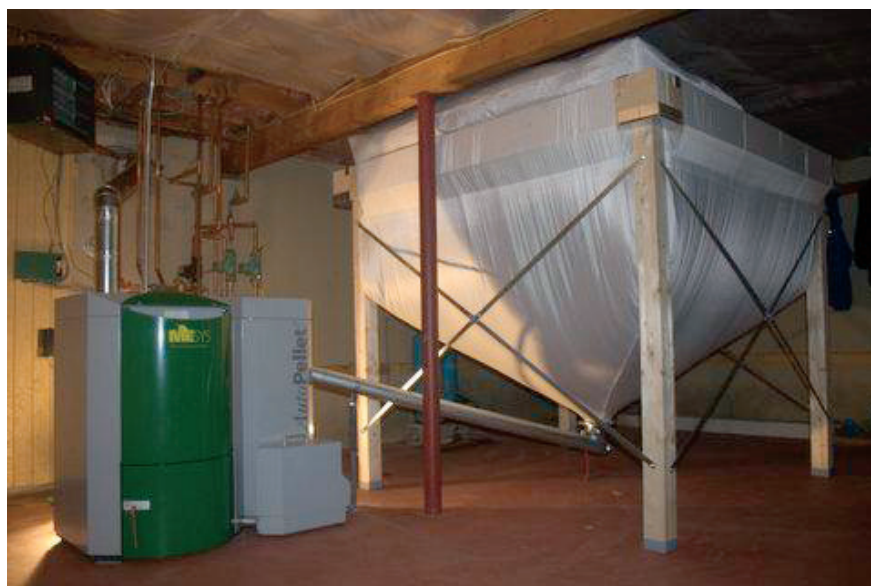
A typical storage bin and wood-pellet boiler. A bin is usually about 6' X 6', about the size of an old coal bin.
