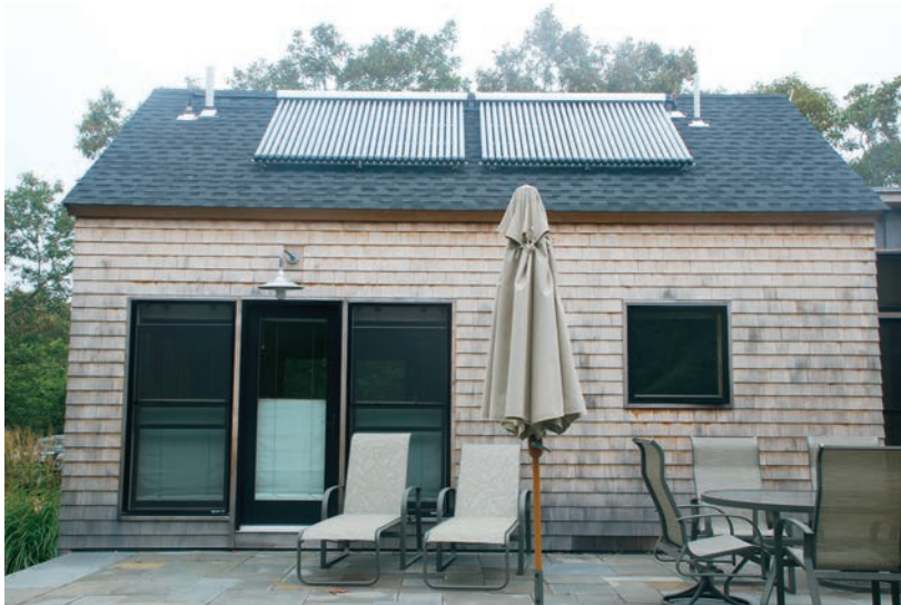
Residential evacuated tube solar domestic water and space heating system on Martha's Vineyard, Massachusetts.
