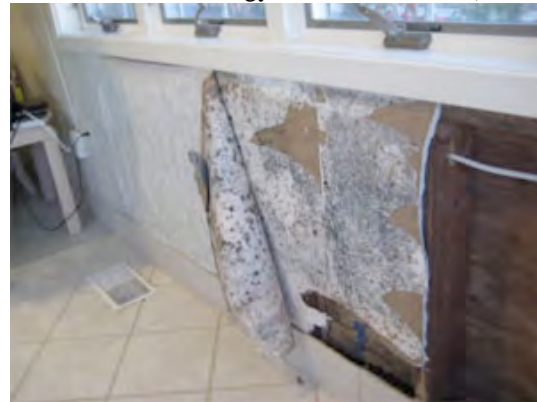
Damage to brick façade of pool building due to lack of proper sealing and air management [Martha Hewett, Minnesota Center for Energy and Environment (MNCEE)]
