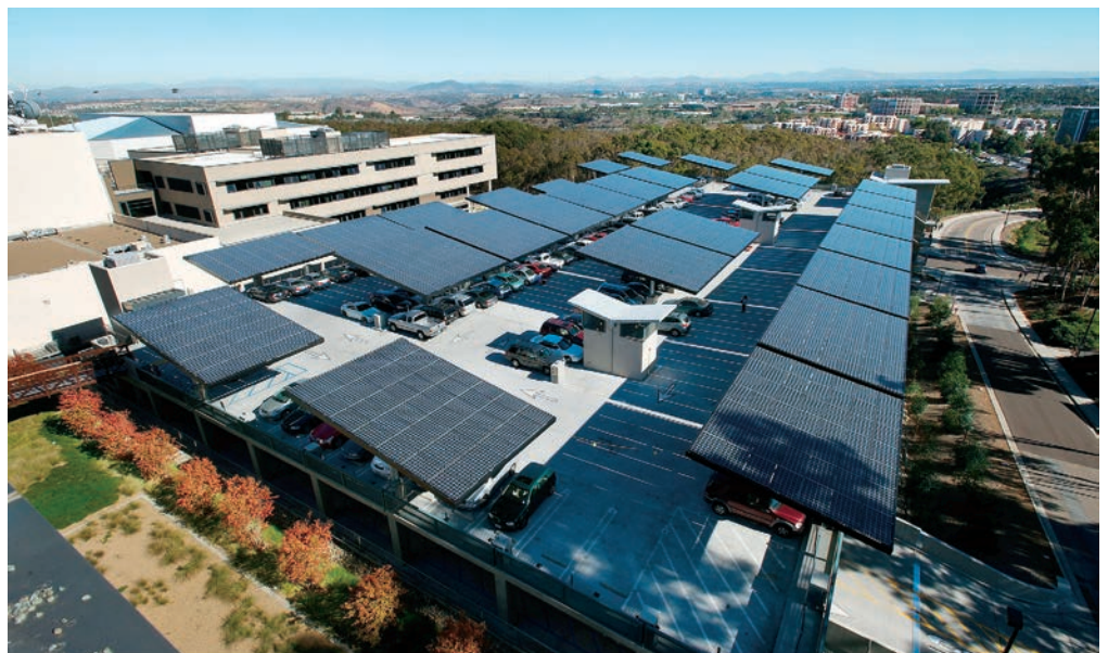
Solar panels provide shade for parked cars and will eventually serve to charge electric vehicles.
