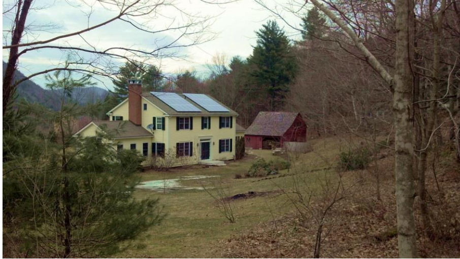
Figure 21: Solar PV Installation in Cornwall, Courtesy of Chris Lenzelec
