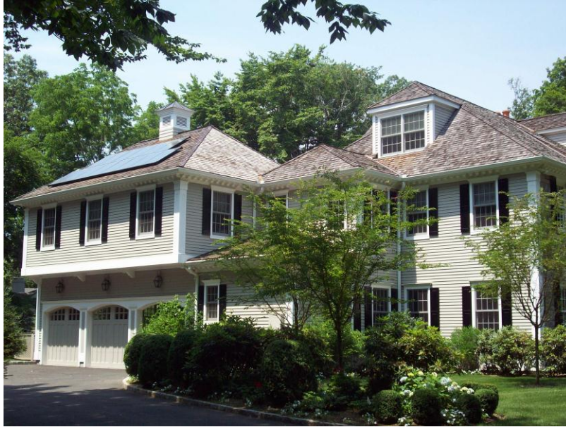
Figure 19: Solar PV Installation in Manchester, Courtesy of Ross Solar Group
