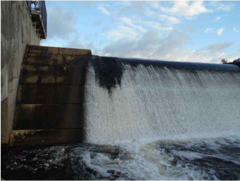
No. 3 Ogee spillway 60 feet long (Spillway No. 1) at the right training wall.
