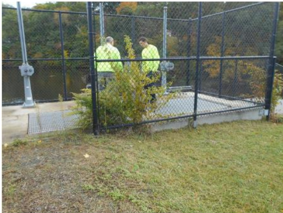
No. 8 Sluice gate operators at the inlet/outlet structure at the right training wall.
