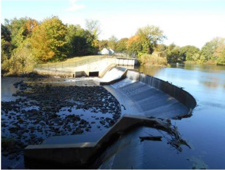
No. 1 Overview of dam from left abutment.
