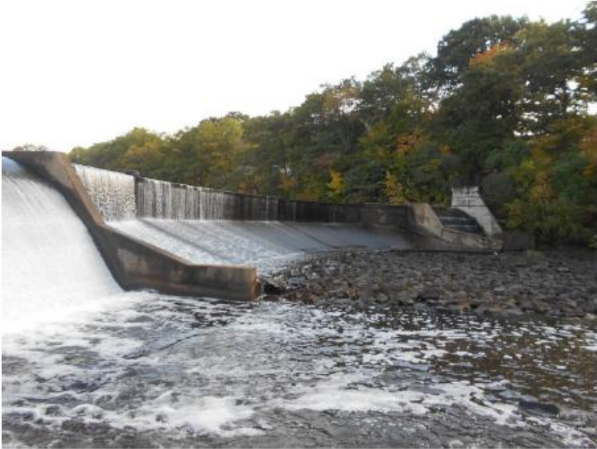
No. 4 Looking from the right at the broadcrested concrete weir center spillway section (Spillway No. 2) 147 feet in length.
