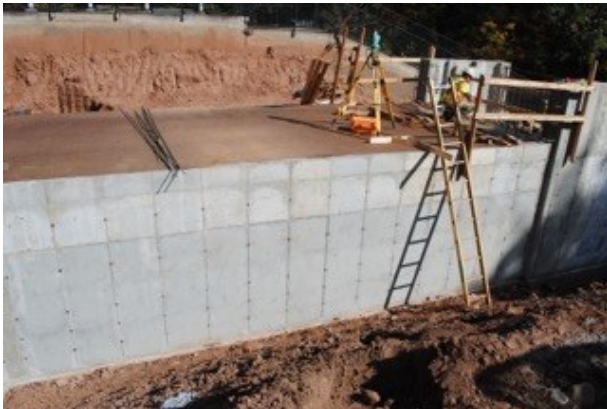
Water intake channel, lateral view
