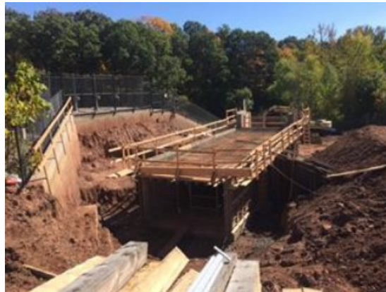
Water intake channel, view from the top
