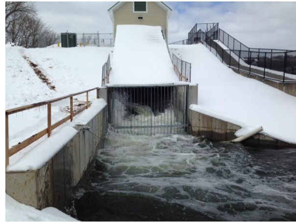
Project completed and operational
